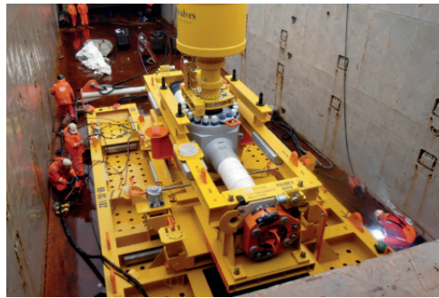
Subsea Riser Positioning
